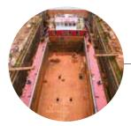
One of the biggest drydocks in Goa's private sector at 84 metres long, 16 metres wide and a draft of 2.5 metres, it has all the necessary infrastructure and facilities to accommodate and repair vessels up to 4000 DWT.
